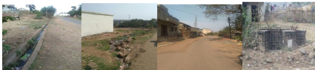
Photograph Various problems in Kandalgaon village
