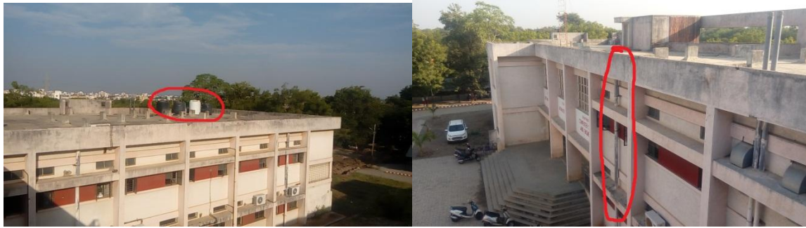
Fig. - 3. Water collection system at Computer Engineering department, Govt. College of Engineering, Amravati
