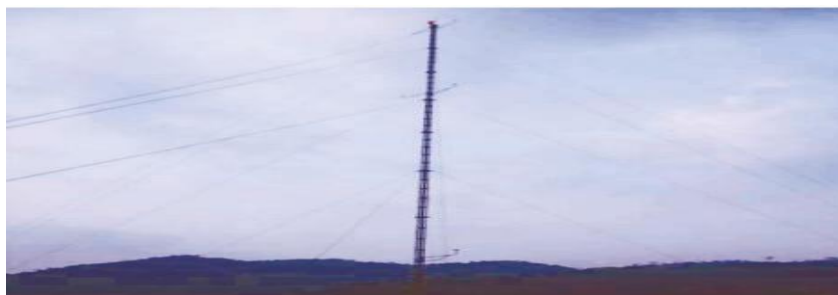
Figure: 3 Wind monitoring station installed at Rombarg, Meghalaya
