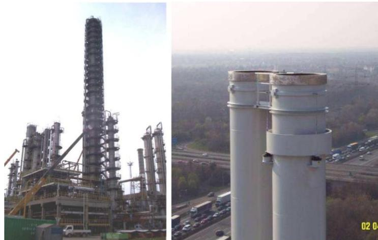
**Fig. 6 Refinery Tower with TMD and Typical Arrangement of Ring Type Systems**
