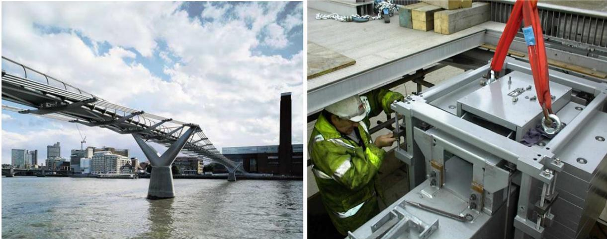
**Fig. 4 Millennium Bridge in London and the Installation of TMDs**
