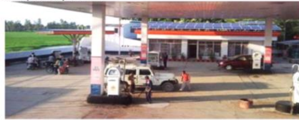
Roof top solar array installation
