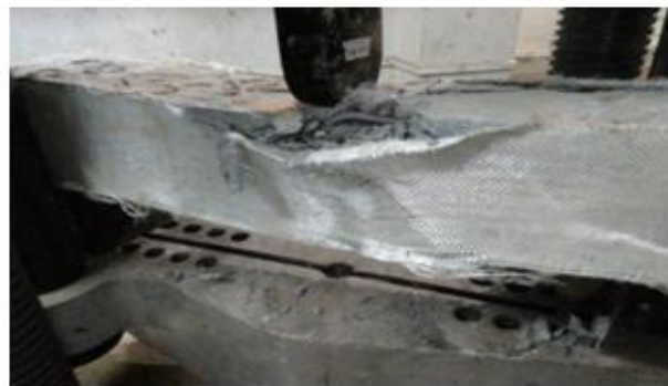
Fig. 5: Failed beam BS2 after testing
