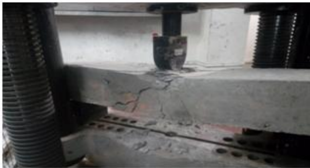
Fig. 1: Failed beam CB1 after testing
