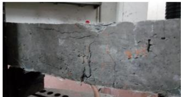
Fig. 14: Failed beam BF5 after testing
