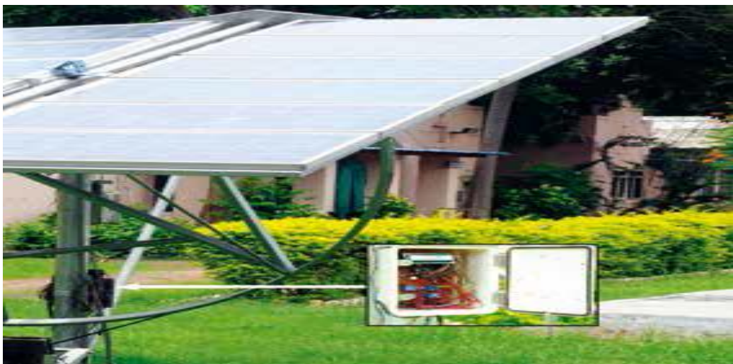
Pic.1: Solar Tracker Mounted with 1kWp PV Modules
