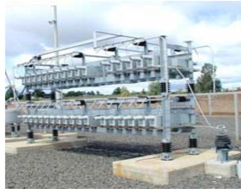
Fig. 9 Block of commercial used capacitors
