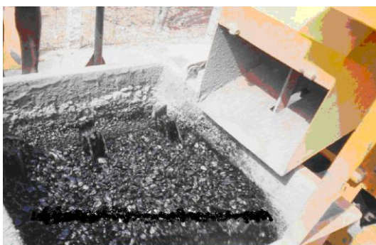
3.1 Hot bitumen is added
