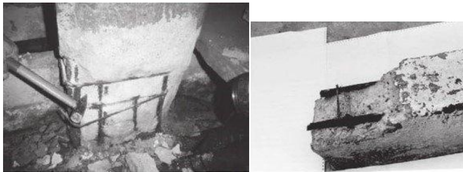
[fig.2 Bamboo Reinforced after 15 yrs exposed to open air]
