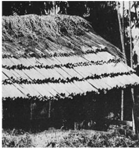
Fig 5(a) Double layers of bamboo shingles
