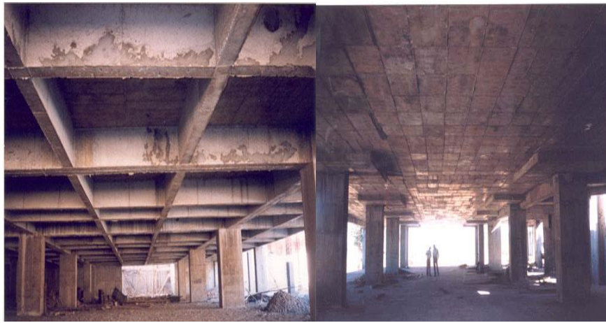
Fig.1 Conventional floor slab system with beam depth
