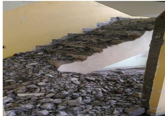
**Fig 2: Demolished Material of Staircase**
