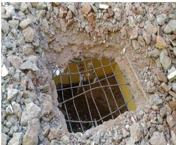
**Fig 3: Central portion of Slab weakening due to Demolition**
